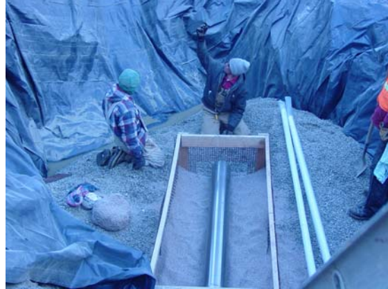
Installation of the intake pipe below the Creek.
